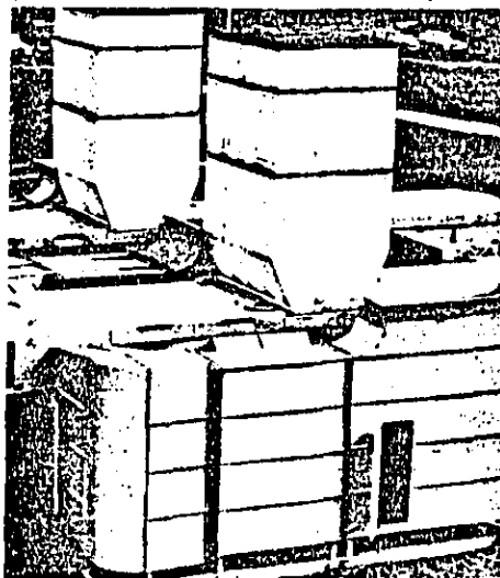
Twin set of gas turbine engines used to generate electrical power. Air intake to engines enters large muffled ducts at each side of engine housing (nearest air inlet duct shown with open access door in foreground.) Engine exhaust gases and noise pass through vertical mufflers in this outdoor installation. (Photograph is courtesy of Diesel and Gas Turbine Progress.)
